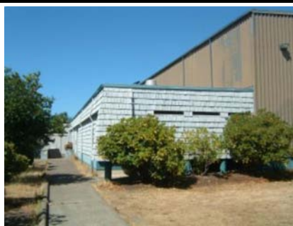
NW Vertical Irregularity Primary primary and secondary structural types also (W2 and S3)
