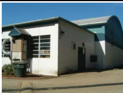
NE Vertical Irregularity Primary reentrant corner also
