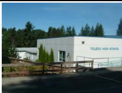
SE Vertical Irregularity Secondary reentrant corner also
