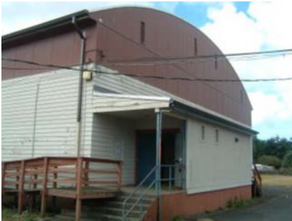
NE Vertical Irregularity Primary reentrant corner also at entryway
