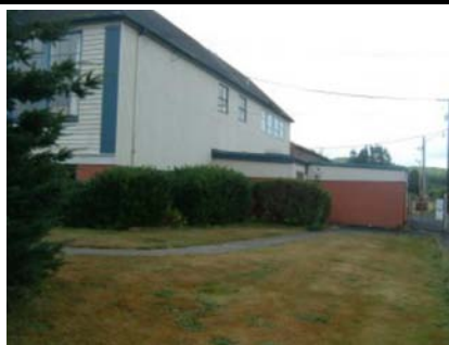
NW Vertical Irregularity Primary reentrant corner also
