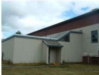
SW Plan Irregularity Primary step in elevation also at the locker room addition
