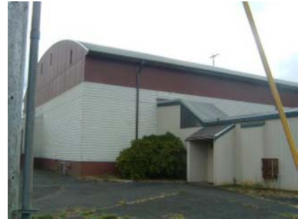
NW Plan Irregularity Primary step in elevation also at locker room addition
