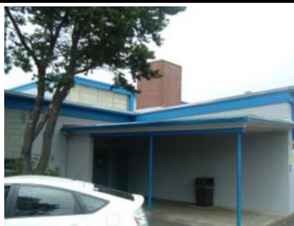
SE Falling Hazard reinforced chimney? Reentrant corner steps in elevation
