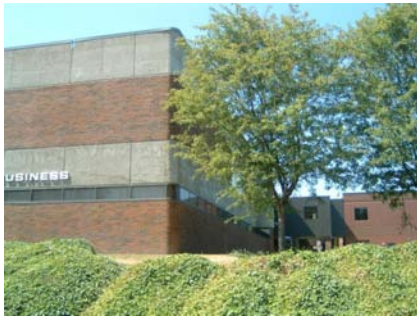
NE General Site
