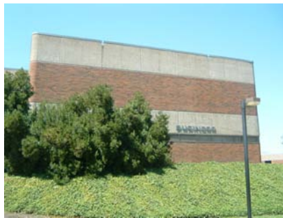
E Falling Hazard
