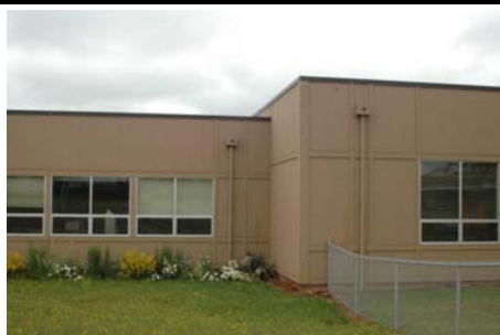
N Vertical Irregularity Primary and plan irregularity - reentrant corner
