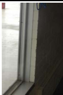
E Primary Structural Type exterior walls are a single course of bricks- compare with image 3
