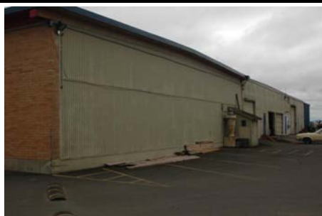
NW Primary Structural Type Brick, wood, and at the far right end light metal.
