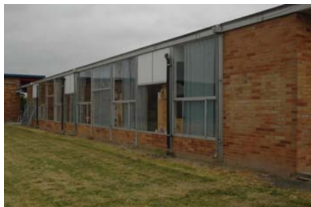
NE Primary Structural Type Other than small masonry end (single course) this wall has wood columns and a lot of glass. Many similar places around school.
