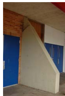
W Other Buttress for glu-lam arch. This is one of the few that are exposed to the exterior. We suspect that the rest land into the main part of the school (n
