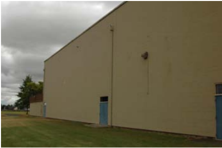
W Vertical Irregularity Primary shorter section on left
