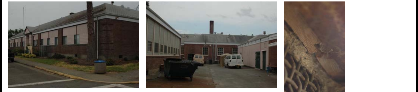
W General Site E Falling Hazard Also shows inside of 'U' W Primary Structural Type Close up from foundation vent. From right to left, metal angle holding brick veneer, the wood tounge and groove. This wood led to the W2 designation.
