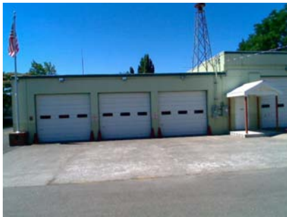
E Primary Structural Type columns on these bays are cast in place concrete, along with the beam above the doors. The rest is RM1
