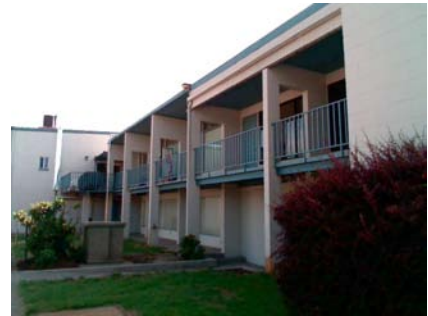
E Falling Hazard CMU BALCONIES
