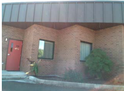
N Plan Irregularity Primary ACCORDION WALLS ON SMALL SECTION
