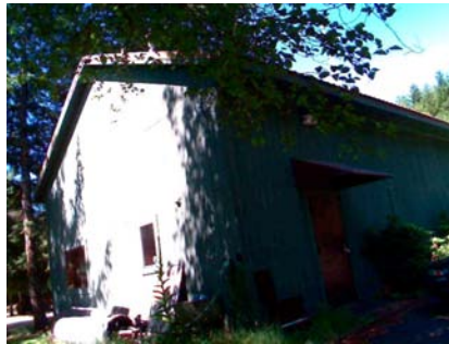
NE General Site
