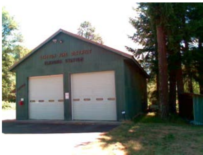
SW General Site
