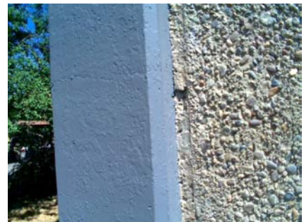
S Primary Structural Type possible tilt up joint.
