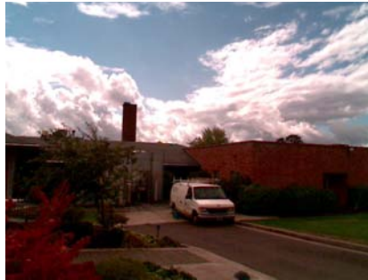
N Vertical Irregularity Secondary ROOF TRANSITION AND CHIMNEY
