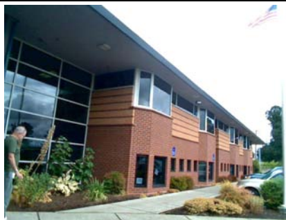
S Primary Structural Type 1993 ADDN IS MOSTLY POLYSTYRENE FILLED W CONC AND BRICK VENEER ACC TO FACILITIES
