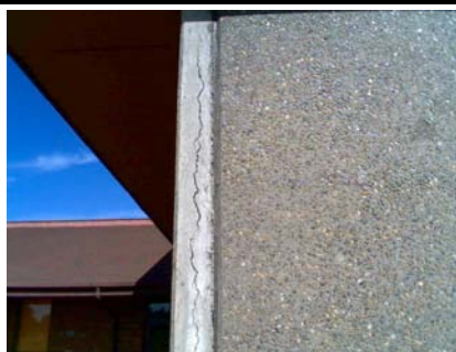
E Poor Condition Tilt up panel has lots of cracks running most of the length of the panel Photos is of cracks on end
