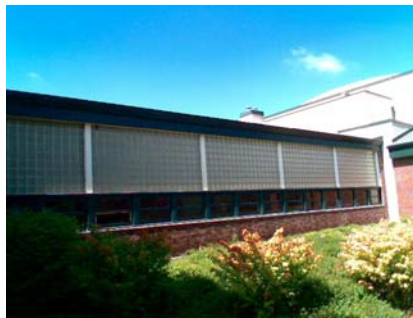
NE Falling Hazard glass block
