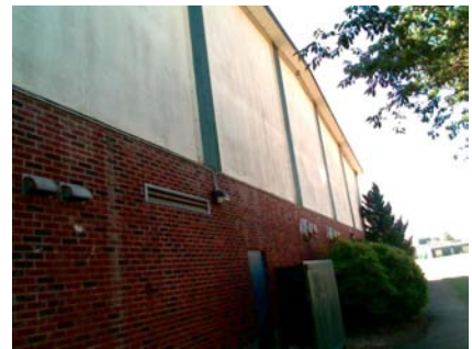
NE General Site plywood siding above brick.
