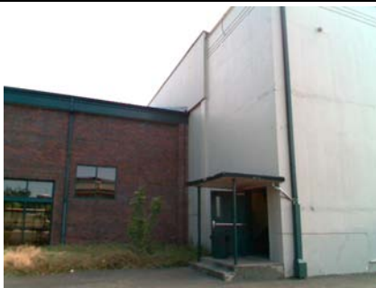
SW General Site new bldg (2000) on left. No visible seismic joint in inside or outside.
