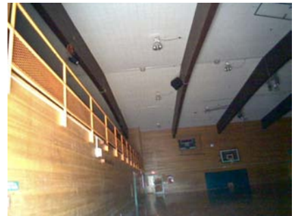
SW Primary Structural Type could not see columns but everything else is wood.
