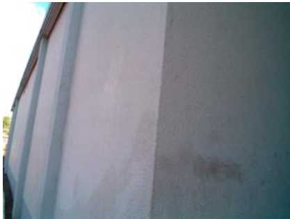
N Primary Structural Type NO CORNER JTS - SO PIP CONC
