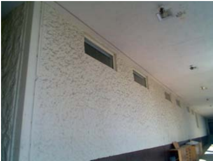
SW Primary Structural Type CONC CAST AROUND STL COLS
