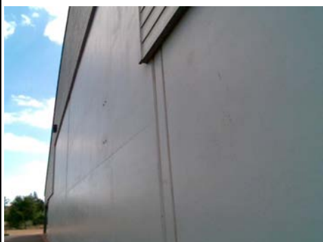
N Secondary Structural Type PC1 ON GYM WALL - THIN MEMB IS STL TUBE COL
