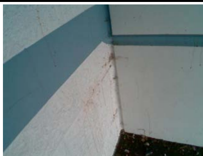
E Pounding Potential Wall on right is PC1 and RM1
