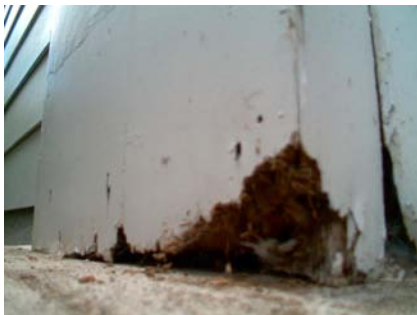
NW Poor Condition Dry rot
