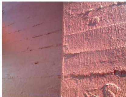
SE Primary Structural Type Concrete form marks.
