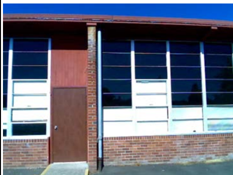
NE Poor Condition brick column shows deflection in middle.
