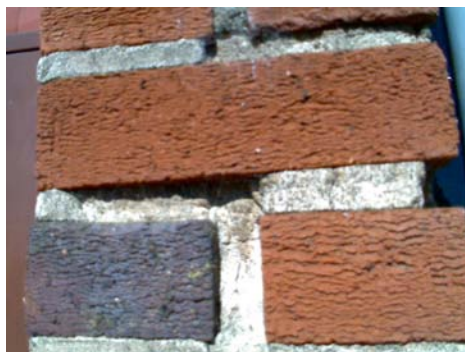
NE Poor Condition middle of brick column. Joint is 1/2" on one side. 3/4" on other. There is a large amount of bowing
