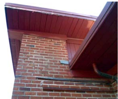
S Primary Structural Type wood walls behind Brick
