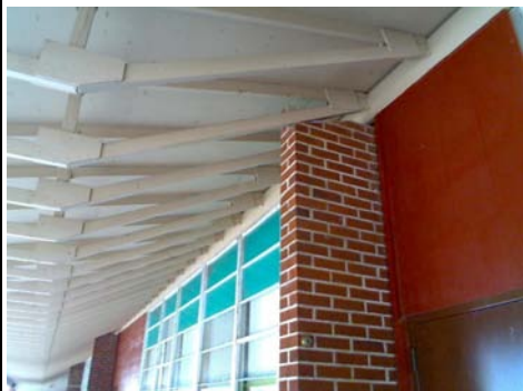
SE Primary Structural Type brick columns are not load bearing on front side (south) of bldg.
