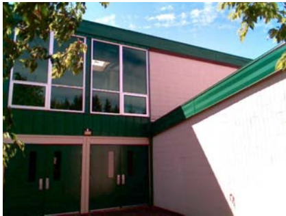
N Pounding Potential bldg D on left and A on right
