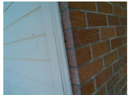
SW Primary Structural Type Wood on left, possible RM1 on right.
