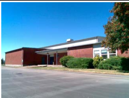
SW General Site
