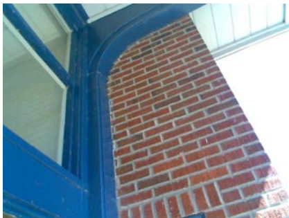
SW Primary Structural Type
