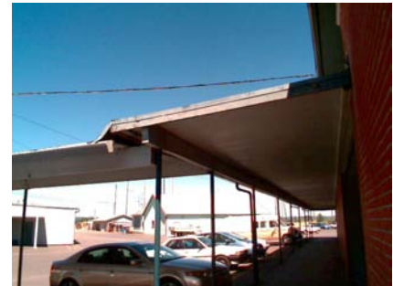
SE Pounding Potential and falling hazard
