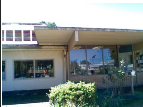
N Pounding Potential bldg B on left A on right.
