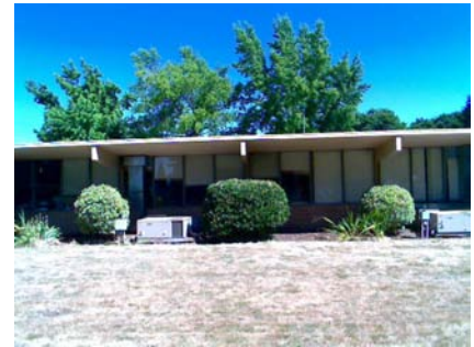
S Primary Structural Type windows go all the way across sides, steel columns between windows.
