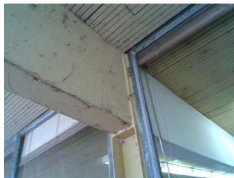
NW Primary Structural Type Top of Column
