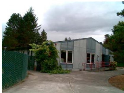
SW General Site Head start bldg too small to screen -2800sqft
