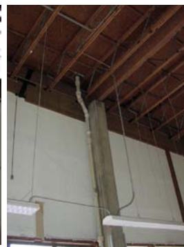
SW Other exterior wall construction from inside
