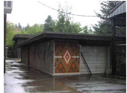
SW General Site small concrete annex
