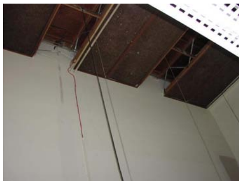
SW Other interior wall
