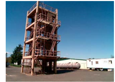
S General Site CONC FRAME TOWER W RM INFILL
