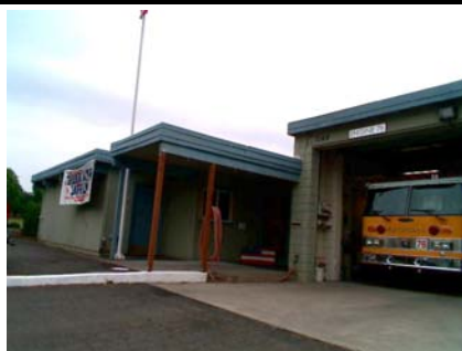
SW Falling Hazard north canopy leg not tied to fdn
