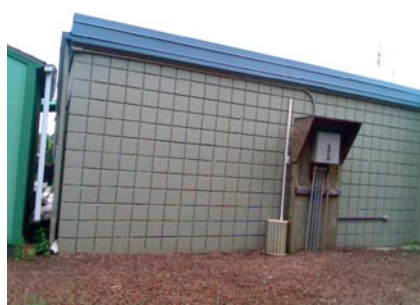
N Pounding Potential between cmu and wood sheds
