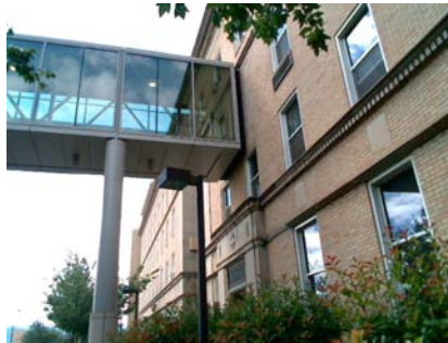
S Other SEISMIC JOINT ON SKYWALK
