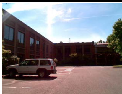
NE Elevation View
