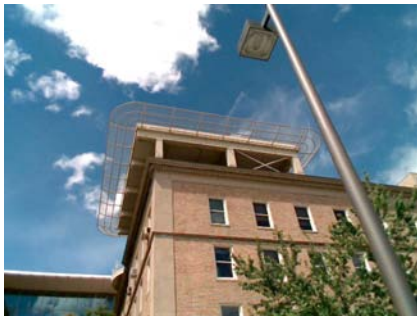
SW Seismic Upgrade
