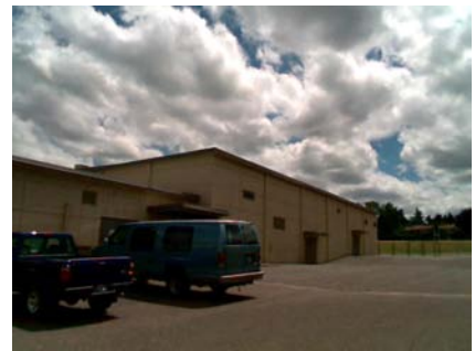
NW Falling Hazard
