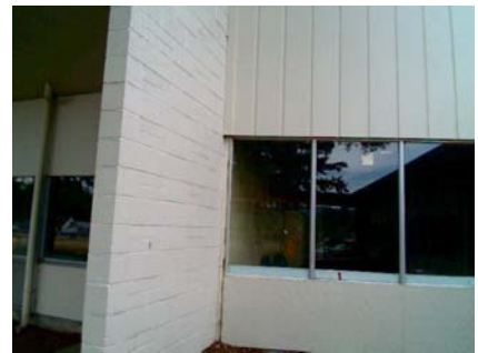
S Primary Structural Type CMU WALL CONTINUES INTO INTERIOR
