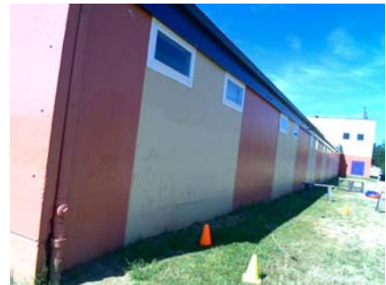
NE Primary Structural Type THIS WALL APPEARS TO BE C.I.P. W/ VERT POUR JTS
