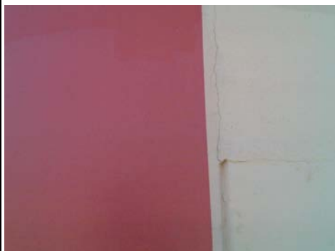
N Primary Structural Type JT DETAIL W/ REVEAL AND VERT (POUR?) CRACK
