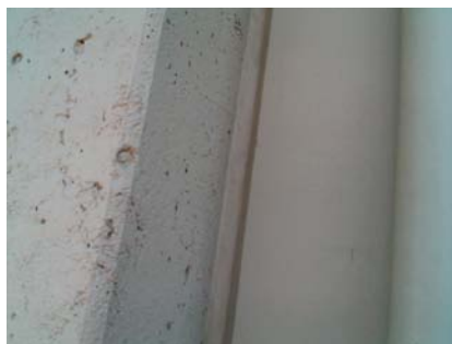
N Secondary Structural Type CAULKED JT BETWEEN D AND C
