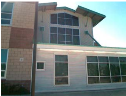
E Primary Structural Type CAN SEE S3 FRAMES IN TALL SPACE
