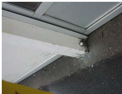
S Poor Condition age of wood column
