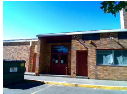
S Primary Structural Type BRICK FIN WALLS ARE 12" WIDE - SUSPECT CAVITY WALL CONSTRUCTION IS HERE - TYPICAL ENTRY DETAIL
