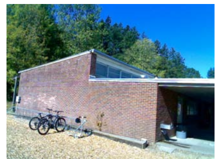
S Elevation View NOTE THICK BRICK ENDWALL ~12"
