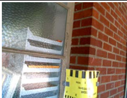
E Primary Structural Type 6" THICK BRICKWORK OUTSIDE JAMB, TOTAL WALL THICKNESS > 12"
