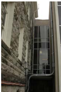
W Other Connection between new building (right) and old URM (left)
