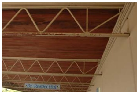
S Falling Hazard concern about how the cover over the walkways is attached.
