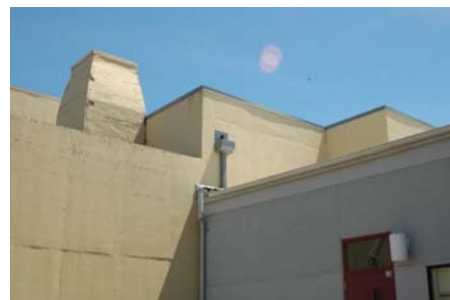
N Vertical Irregularity Secondary Also shows a plan irregularity due to an adjacent building. Building B is on the left and building A is on the right.
