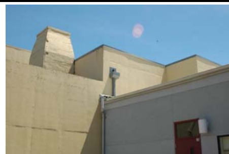
NW Vertical Irregularity Secondary Building B is on the left and building A is on the right.
