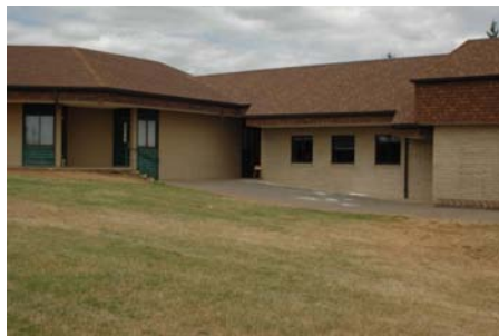
SW Vertical Irregularity Primary steps in elevation also, and reentrant corners
