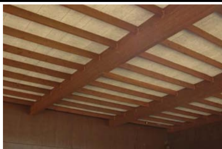
N Secondary Structural Type wood beams in roof
