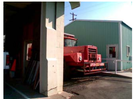
S Poor Condition pier cracks
