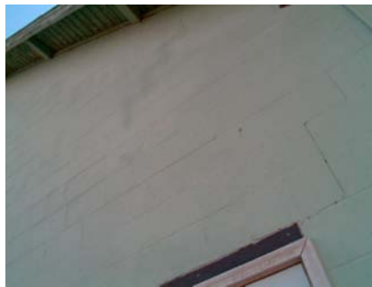
W Building Quality stairstep crack
