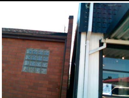
N Pounding Potential NO POUNDING, 6" GAP
