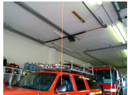
N Primary Structural Type PILASTERS
