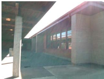
NW Seismic Upgrade BUTRESSES
