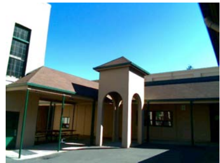
N Falling Hazard cmu feature
